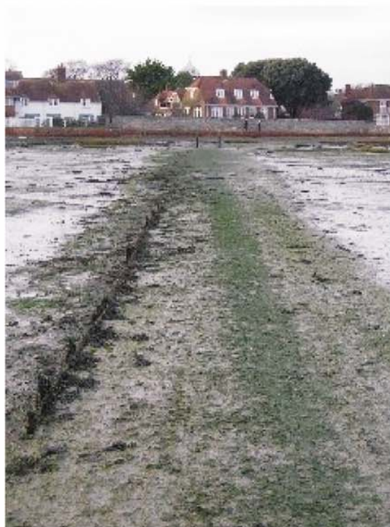
Fig 19 The Wadeway between Langstone and North Hayling, looking north (photo MoLAS). Timber structures can be seen on the left of the image
