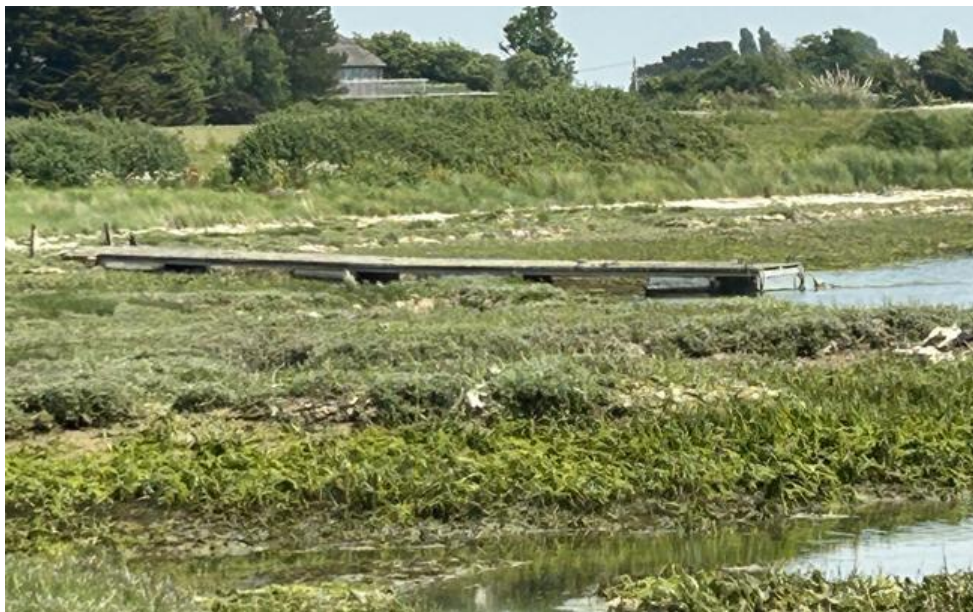
Figure 2 Existing pontoon in situ
