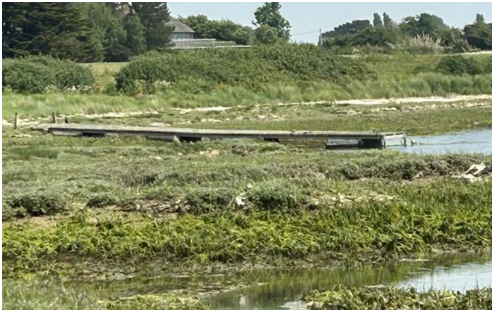
Figure 2 Existing pontoon in situ
