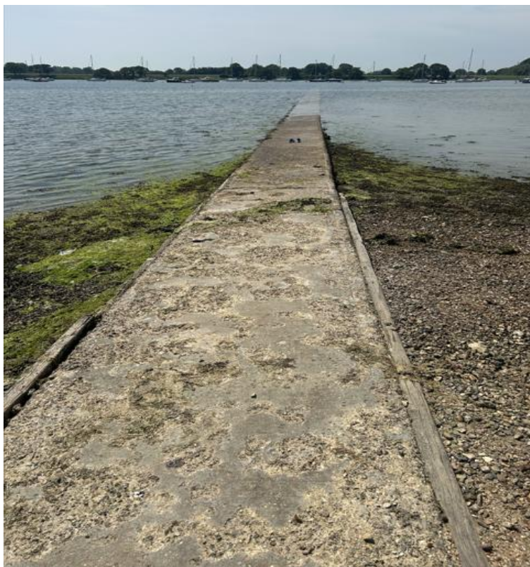
Figure 4 Landward end of the Hard showing part of the gravel to be replenished.
