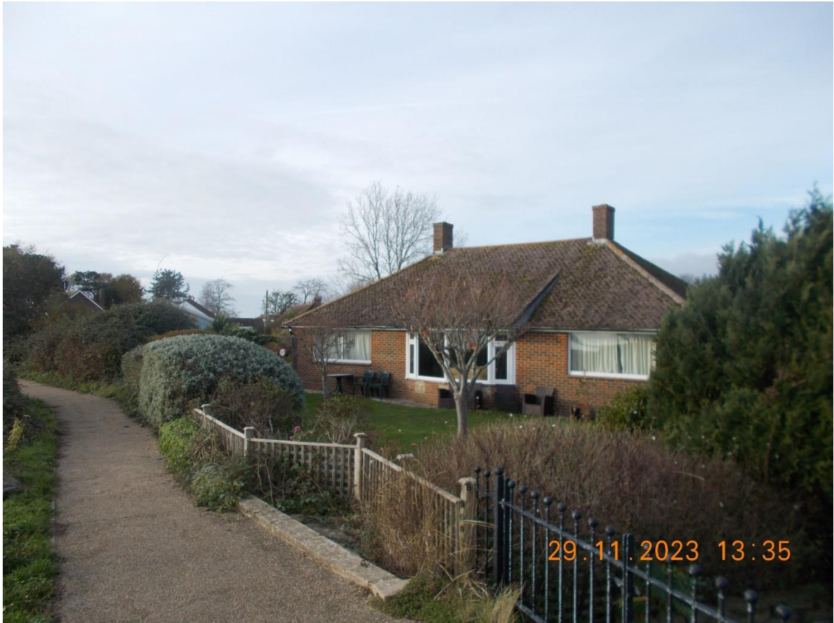
Existing south elevation (view from foreshore seawall footpath)
