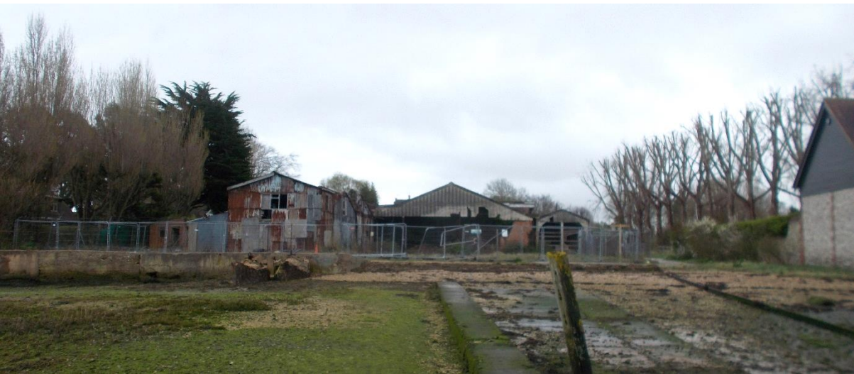
Above: View from concrete jetty/slipway in front of site
