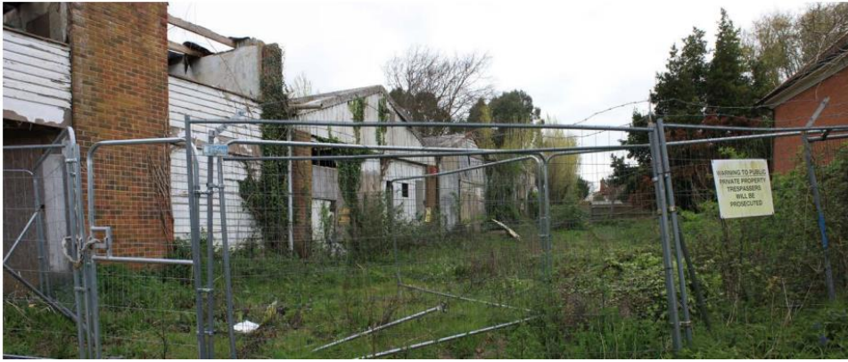
Above: View from footpath to south of site
