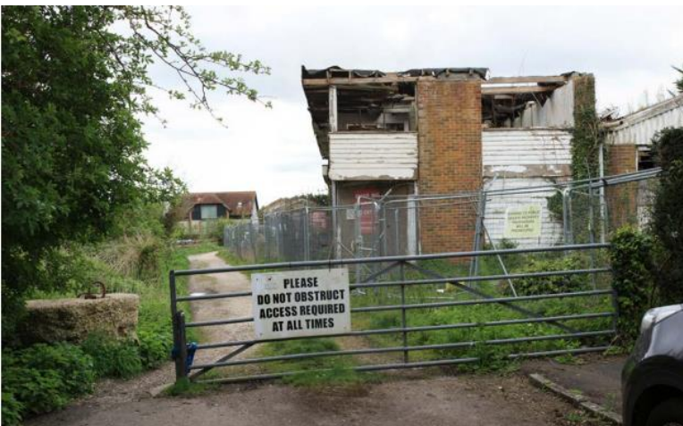
Above: View from footpath to east of site
