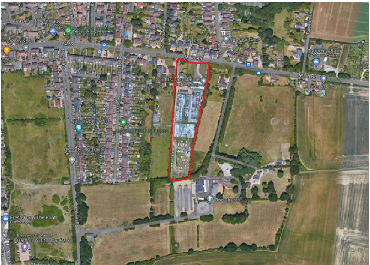
Above: aerial photo showing location of the site
