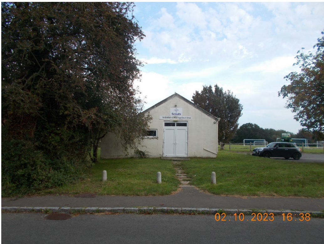
Above: View from Crooked Lane of front of building.
