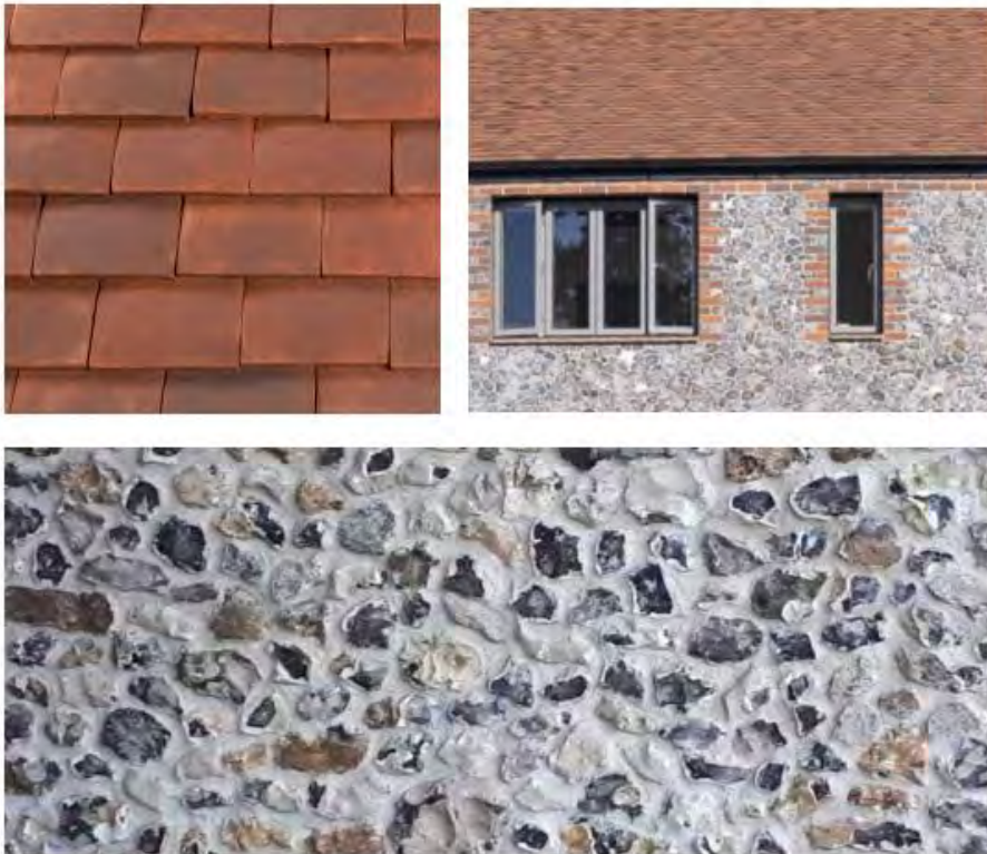
HANDMADE CLAY TILES FIELD FLINT SOURCED LOCALLY WITH RECLAIMED BRICK COINING AROUND OPENINGS
