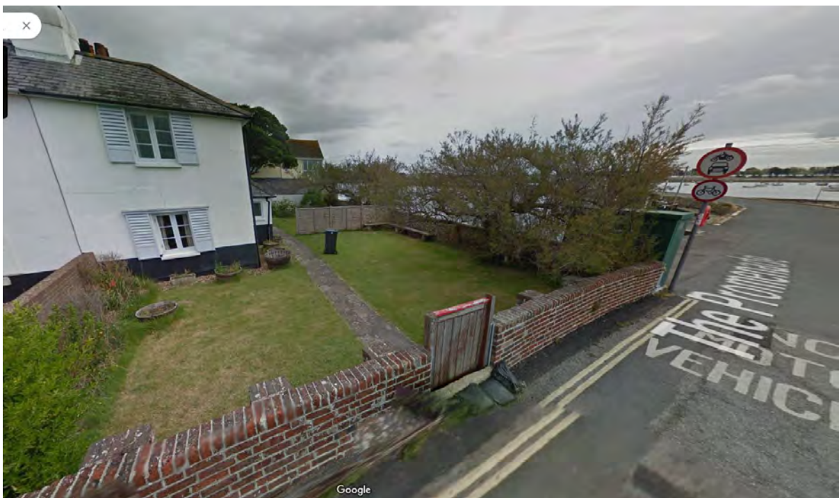
Above: Existing southern boundary wall and gate to property opposite the proposed new wall
