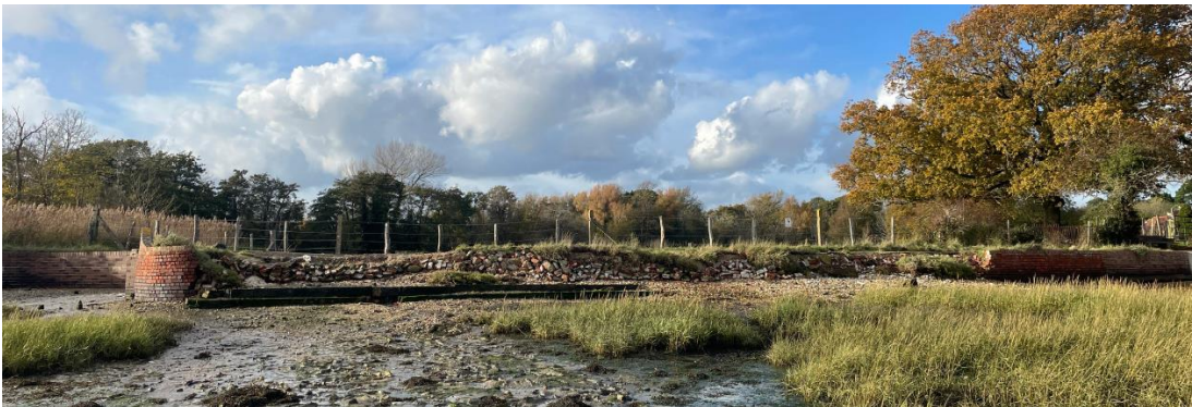
Figure 2. Present day view of sea wall.
