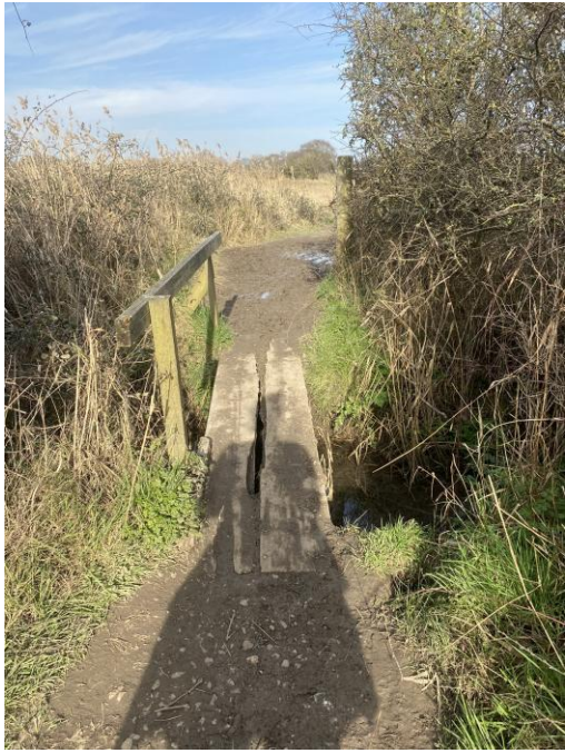
Figure 3 Footbridge to be replaced.
