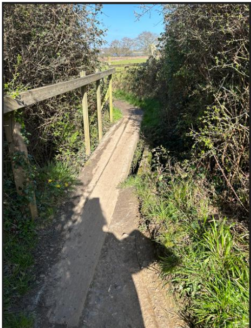
Figure 4. Footbridge to be repaired.
