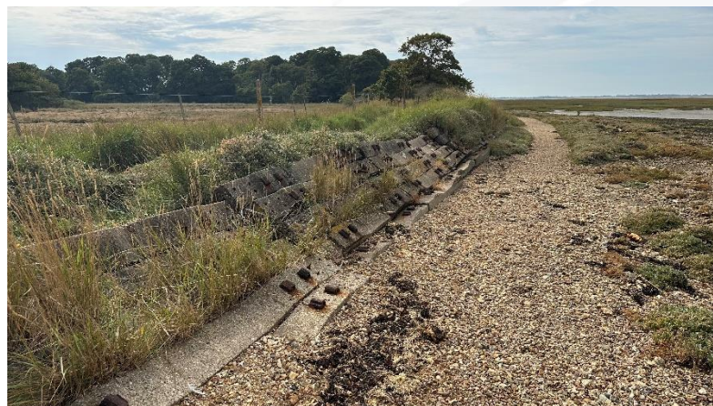
Figure 2: Old defences concrete sea defences at Chalkdock Marsh.
