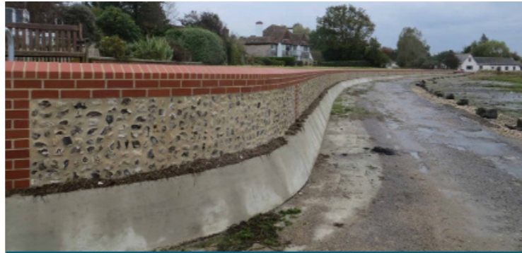
Solid wall protecting property at Bosham
