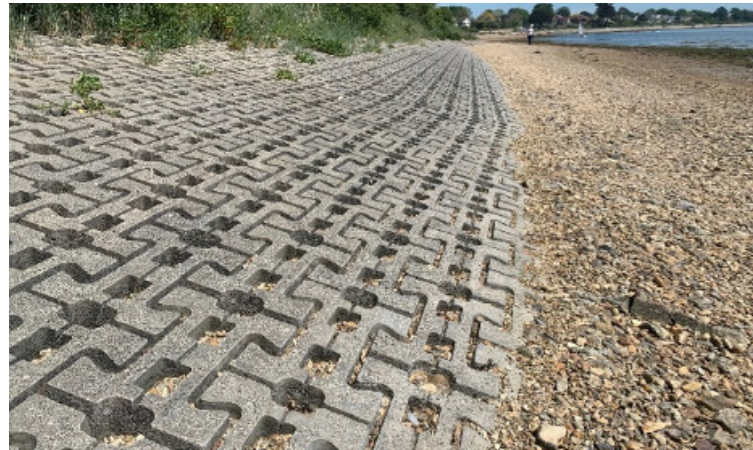
Concrete revetment at Nore Barn woods
