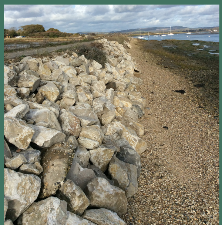
Rip-Rap sea defence in Chichester Harbour
