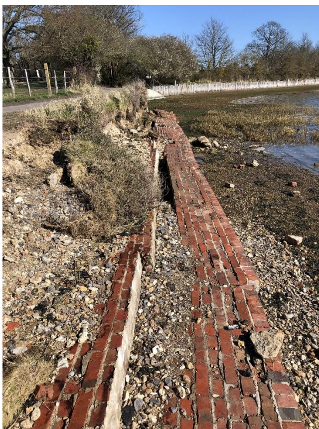
View looking north near "FB", collapsed sea wall in foreground, timber piles in distance.
