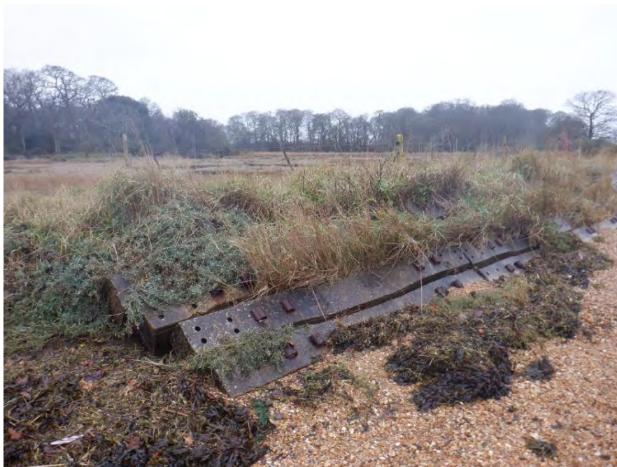
Figure 3.11. Eastern end of the protected frontage with seaweed present at the toe of the structure.
