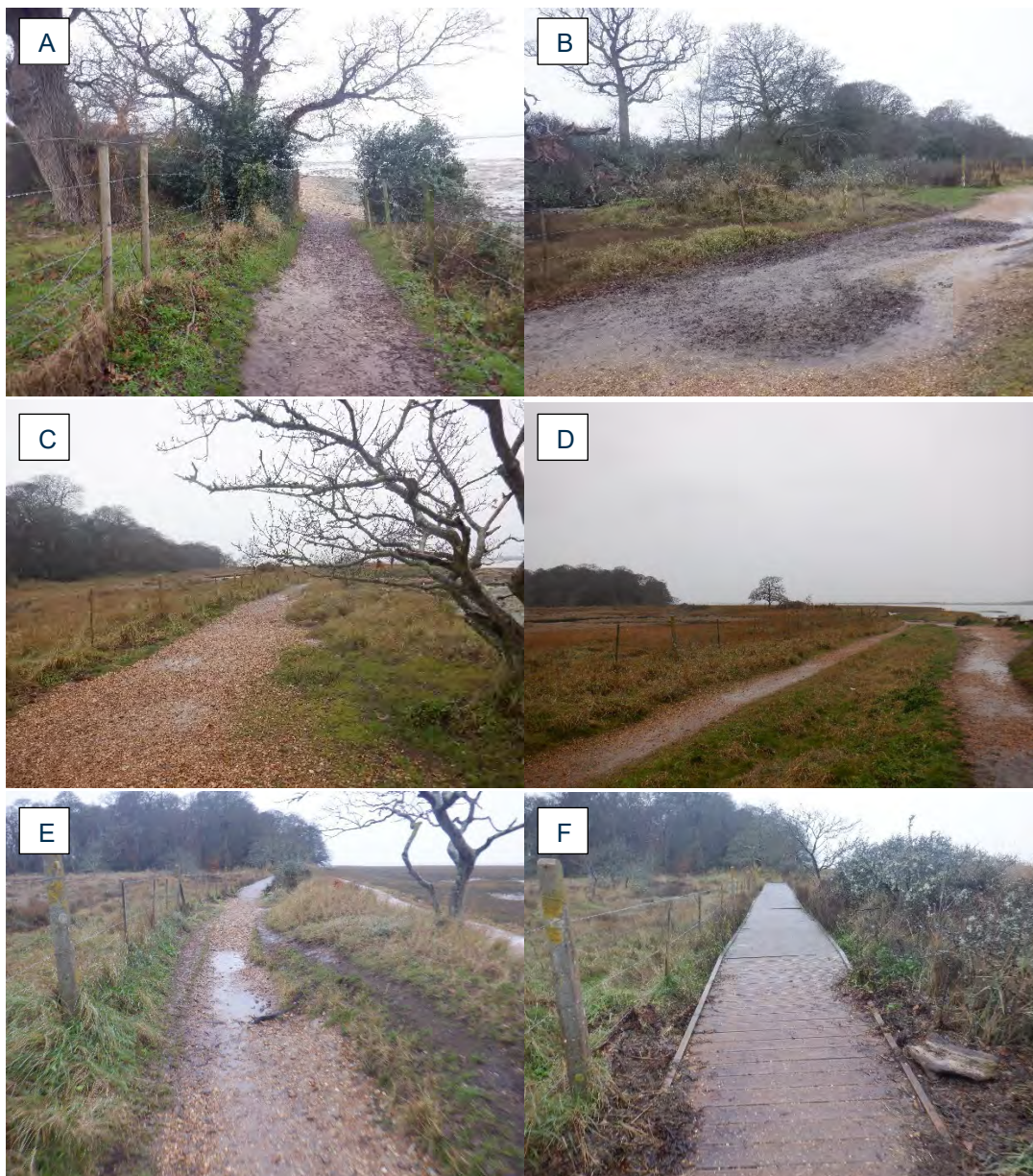
Figure 2.1. Footpath condition, with photos from A to F showing the conditions from the east to west of section WEI-1.
